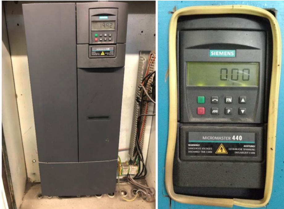
**Figure 20.** Frequency converter Siemens Micromaster 440
